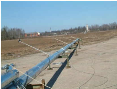
Fig. 5. Installation of the 60-m high mast with a measuring complex Symphonie 9200 together with sensors on metal 1.8-m long mounting boom (site 2).
