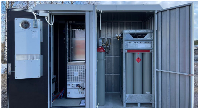
Fig. 6. The chosen system's 5 kW outdoor installation with external hydrogen bottles.
