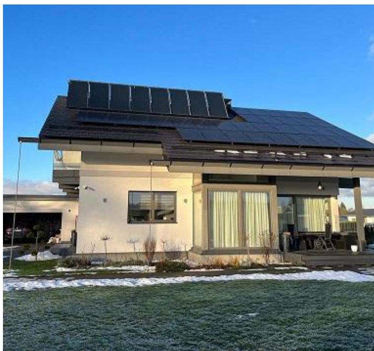
Fig. 1. Solar collectors and photovoltaic panels on the roof of the building.
