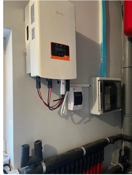
Fig. 3. Solar inverter and control unit.
