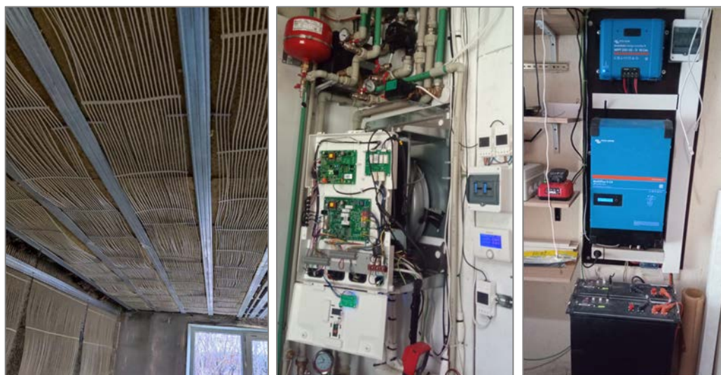
Fig. 3. The main used components – capillary mats, heat pump and battery (see also Fig. 4).
