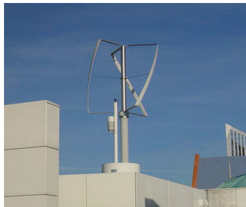
Fig. 3. Vertical Axis Wind Turbine (VAWT) Darrieus H-type 0.75 kW.
