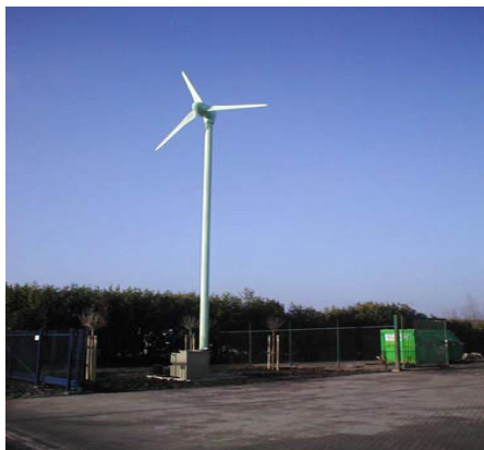
Fig. 2. Horizontal Axis Wind Turbine (HAWT) 0.75 kW.
