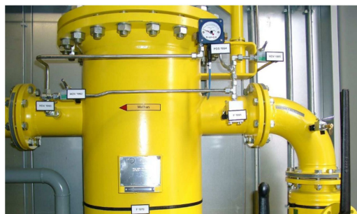
Fig. 2. Biomethane piping and measurement equipment in the grid connection station, Germany.
